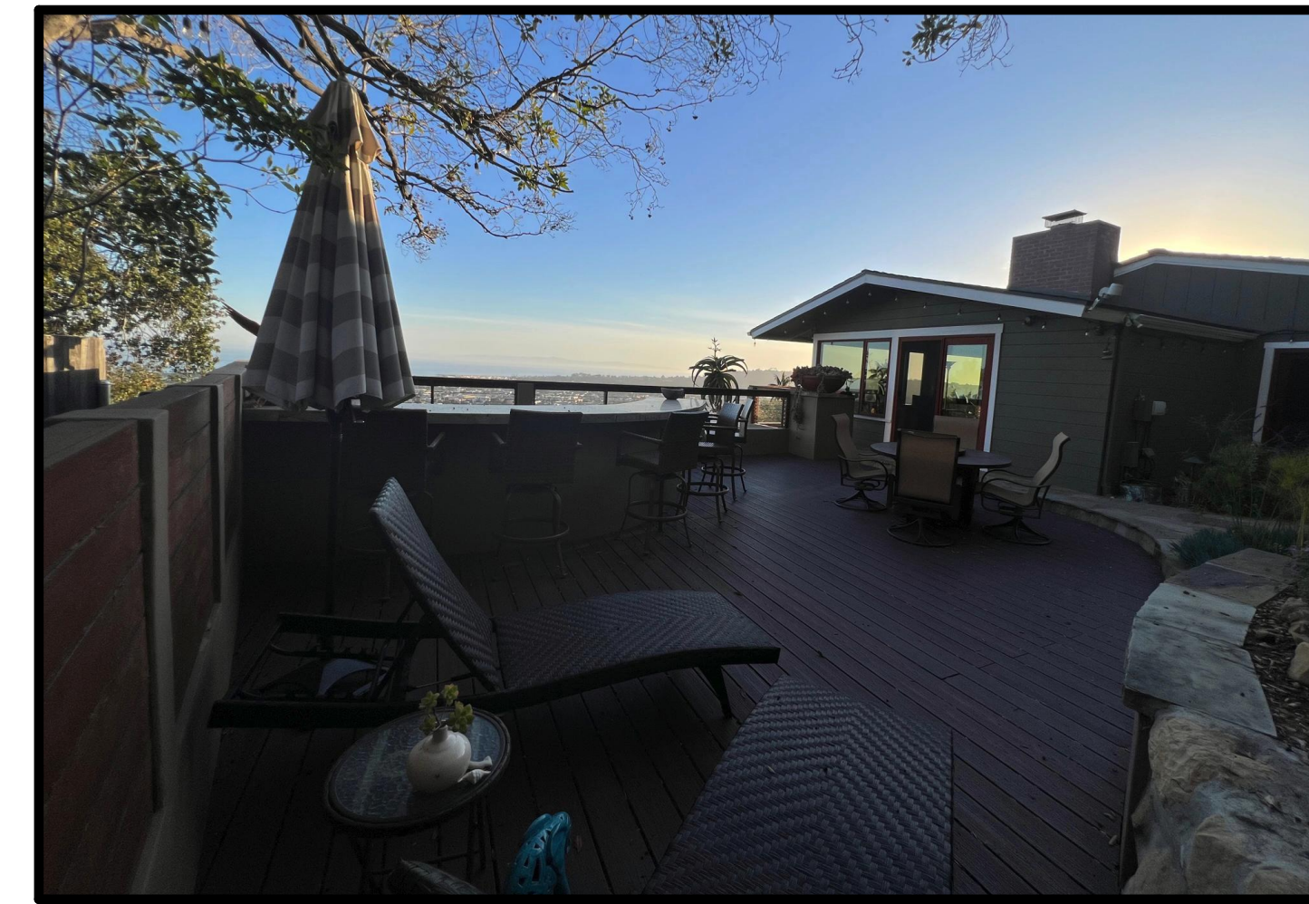
EAST FACADE - MAIN RESIDENCE
